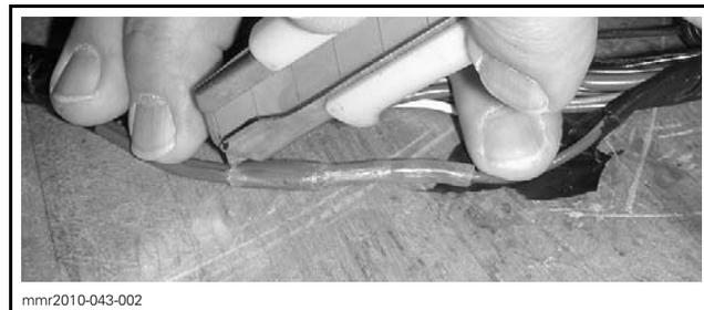
**NOTICE** Be careful with the blade to avoid cutting wires insulation.
